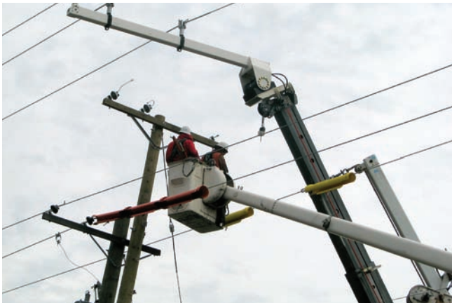
Live Line Solution's Insulated Conductor Support Jibs (ICSJ) and LinePro HA keep linemen safe and increase productivity by incorporating radio-controlled, hydraulic-actuated articulation.
